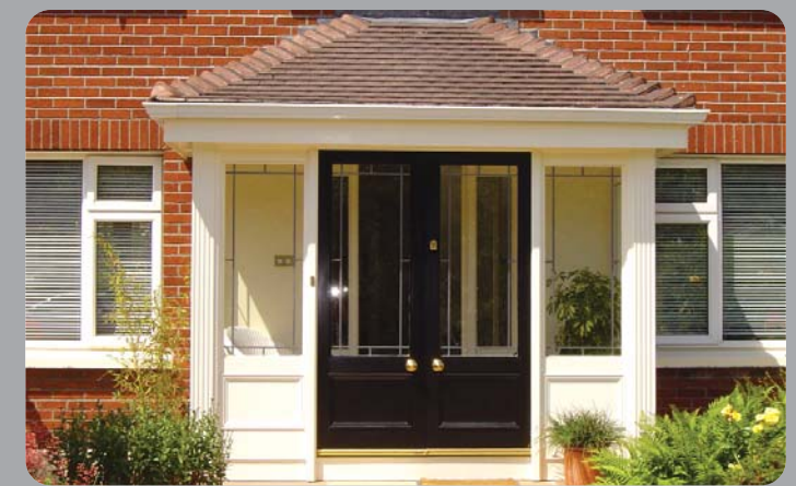
Porch supplied by McNally Joinery
