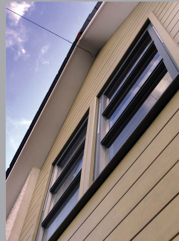
World's first Accoya® clad house
