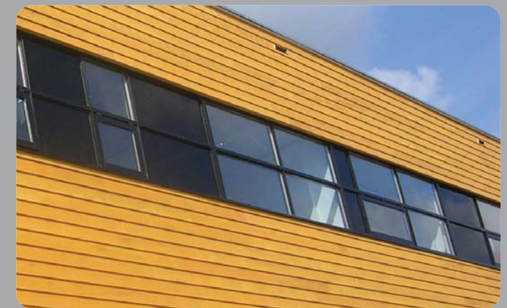
Accoya® cladding with translucent wood stain coating on MP4 building
